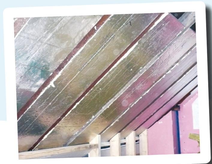
*Sloping ceiling insulation being installed between rafters*
