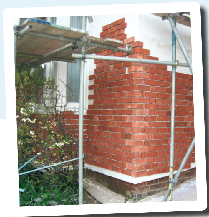
Brick slip being applied to insulated walls
