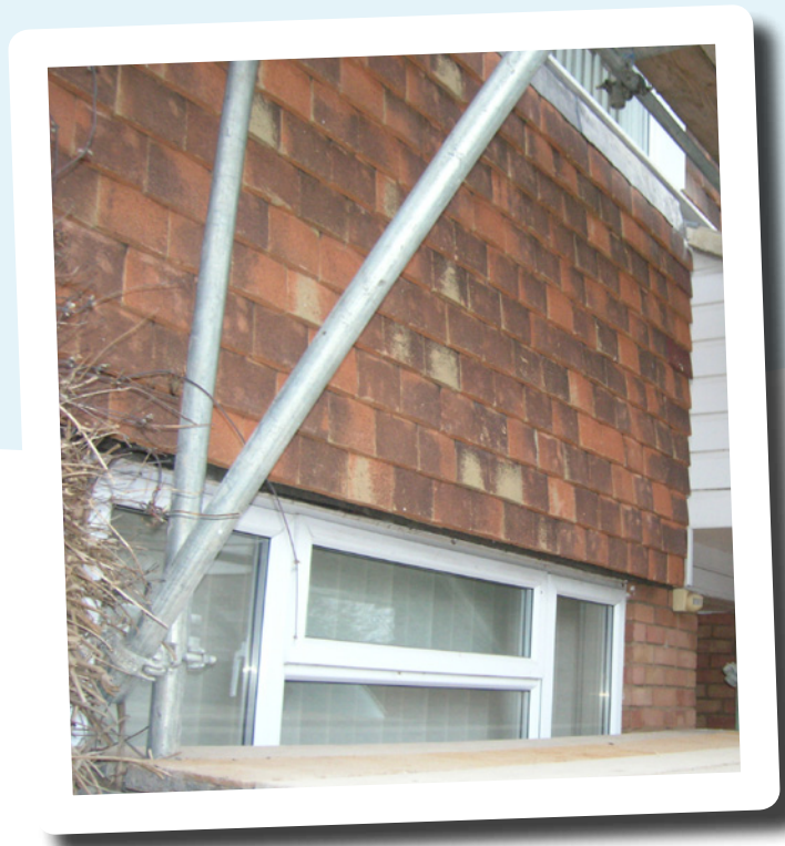
Tile hung wall after insulation installed
