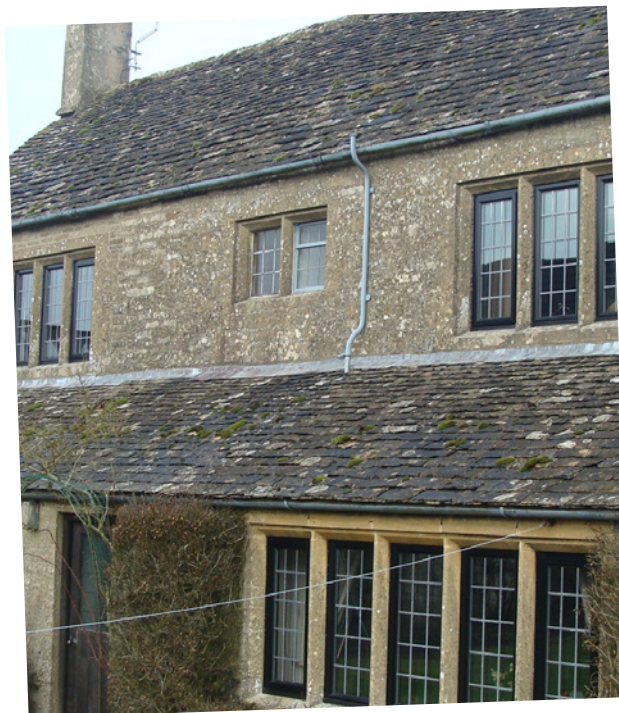
New double glazed windows at rear of property
