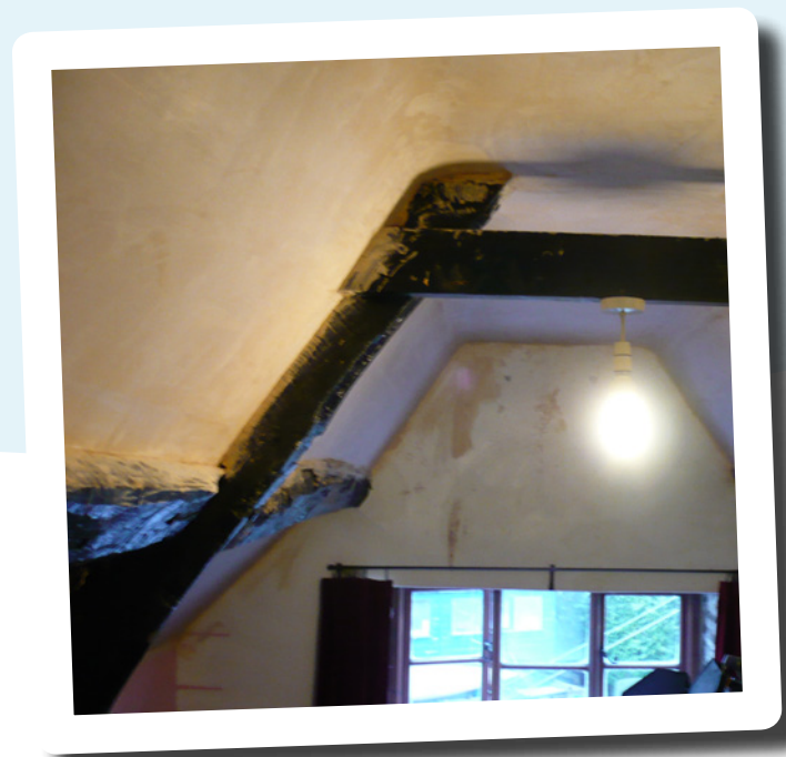
Completed sloping ceiling insulation re-plastered and ready for redecoration
