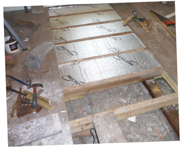
Installing insulation below floor boards
