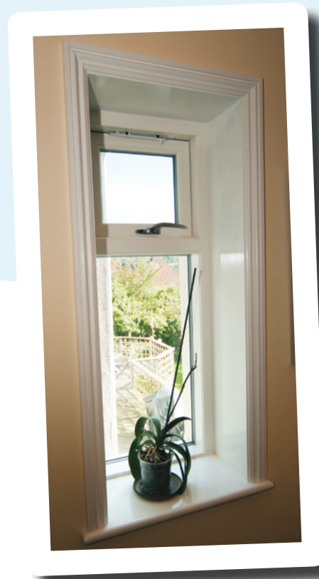
Finished internal wall insulation and new high efficiency window
