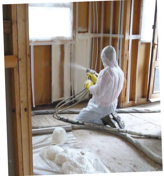
Spraying foam insulation into timber frame walls
