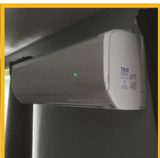
Air to air heat pumps to replace old oil system
