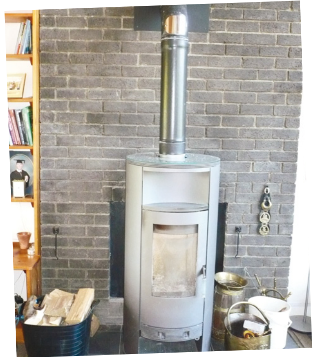
High efficiency woodburning stove
