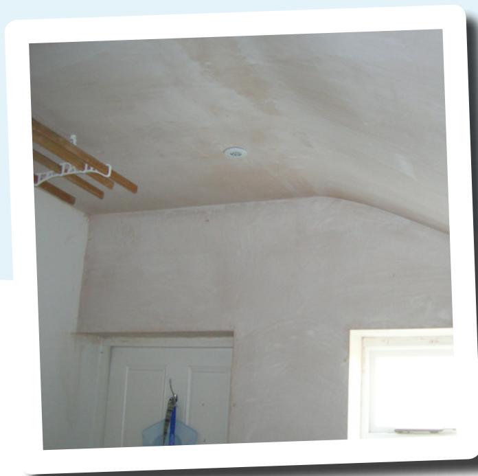
Insulated walls and ceiling ready for redecoration
