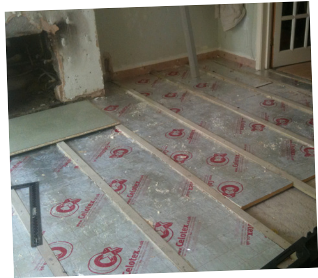
Installing underfloor insulation in living room
