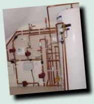
Ground source heat pumps (GSHPs) also work on the vapour compression refrigeration cycle principle, but can typically offer higher efficiencies than air source systems by using year-round low-grade heat from the ground.
