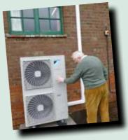
Air-to-water heat pumps are an alternative to air-to-air systems, although they work on the same principle.
