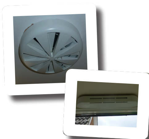
Passive ventilation system - ceiling and window vents
