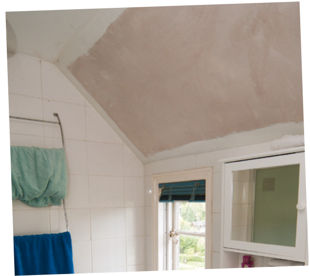
Sloping ceiling insulation ready for decoration
