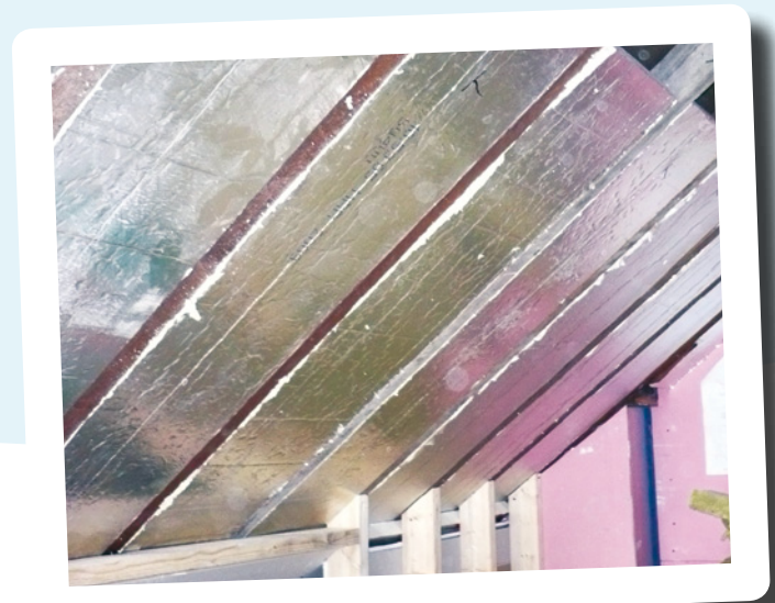
Sloping ceiling insulation being installed between rafters
