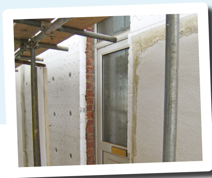
Insulation boards applied and render in progress
