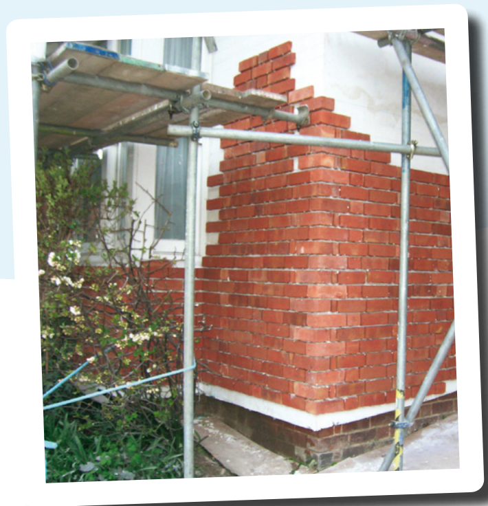
Brick slip being applied to insulated walls
