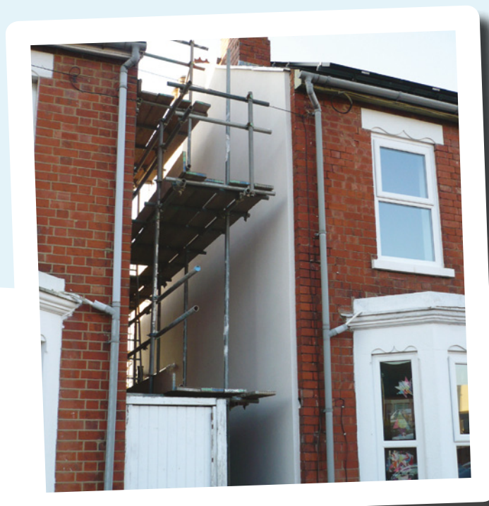
The final coat of render being applied to insulated side wall
