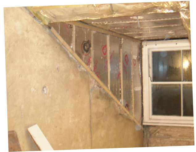
Insulation in progress to the bay window and sloping ceiling
