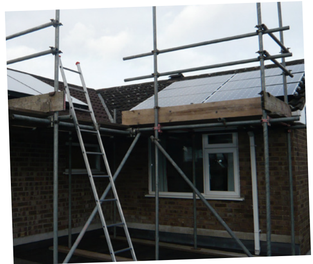
PV and solar thermal panels mounted on south east and south west facing roofs
