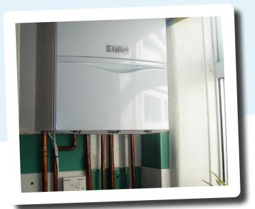
Back boiler replaced with combi boiler mounted on the kitchen wall
