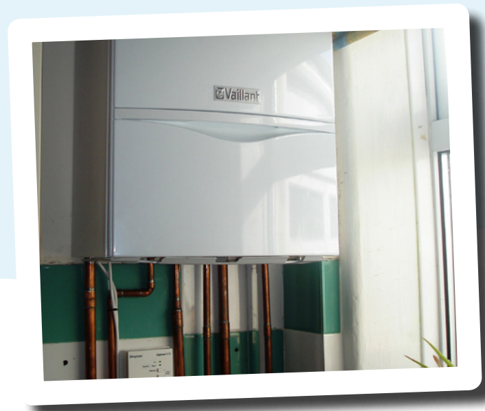
Back boiler replaced with combi boiler mounted on the kitchen wall
