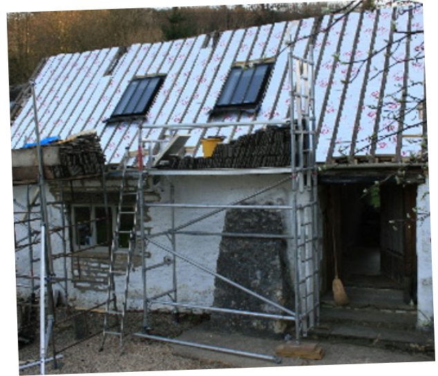
Insulation installed between rafters after removing roof tiles
