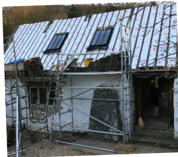
Insulation installed between rafters after removing roof tiles
