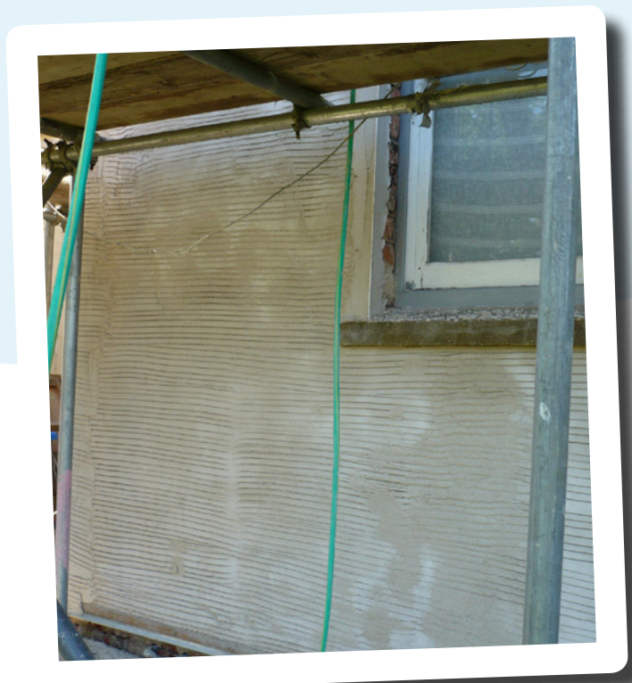
Applying insulating lime render to rear wall of house
