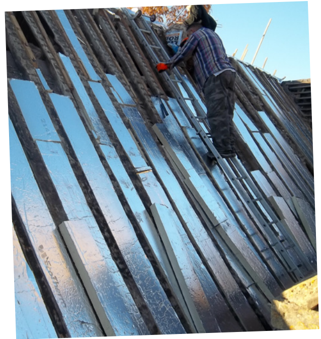
Installing sloping ceiling insulation between rafters after tiles removed
