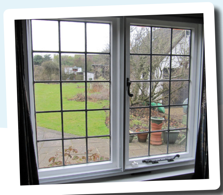
Unobtrusive secondary glazing installed behind single glazed window
