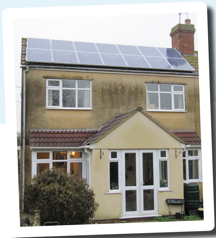
Completed PV installation on south facing roof
