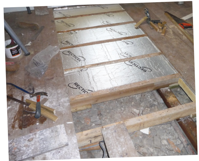
Installing insulation below floor boards
