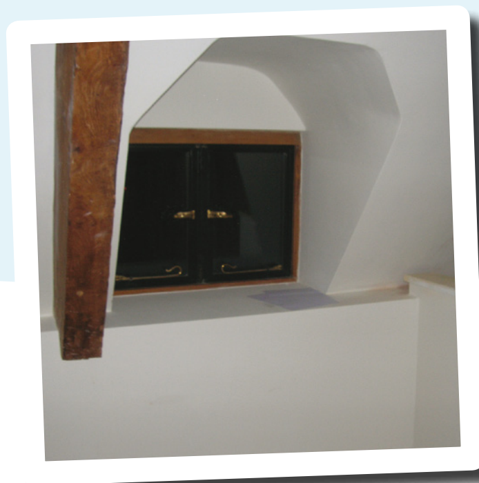
Insulated walls finished in keeping with character of the cottage
