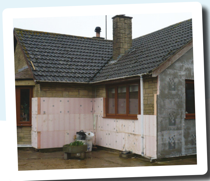
Installing external wall insulation
