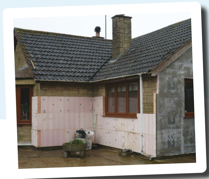
Installing external wall insulation
