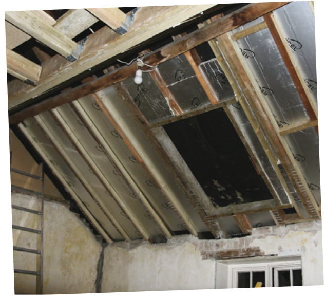
Sloping ceiling insulation being installed
