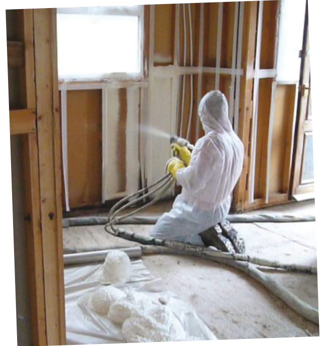
Spraying foam insulation into timber frame walls
